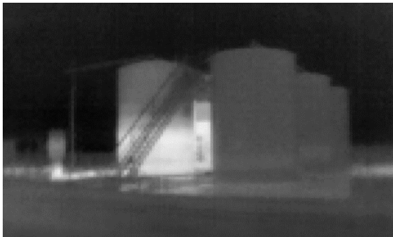
Tank battery fuel levels can be determined from a safe distance with thermal imaging.
